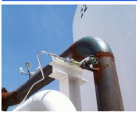
D-2 Incorporated has developed an additive injection quill for the fuel industry. These injection quills can be built with either a retractable mount assembly or fixed position assembly.
